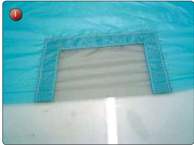
10. Draw a line along the edge of the partial panel on each side from the point where the old panel meets the new one. Trim the fabric along this line. [Figure J]
