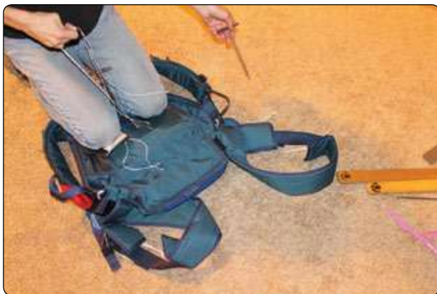
Figure 5-160. Pull the bodkins with their respective pull up cords through the pack.
